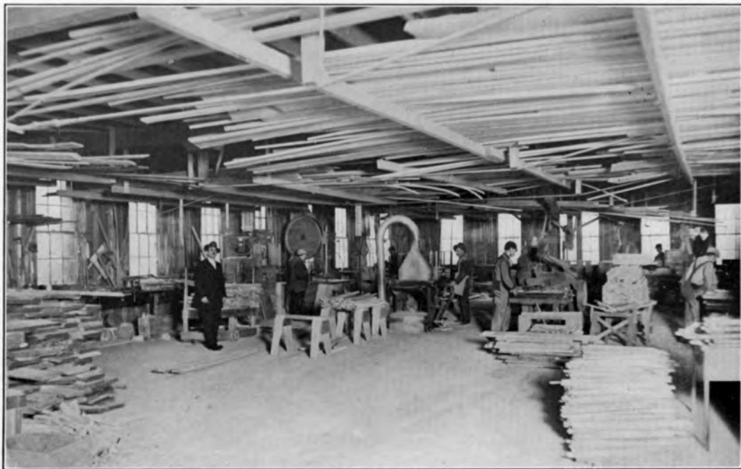
WOODWORKING MACHINE ROOM
