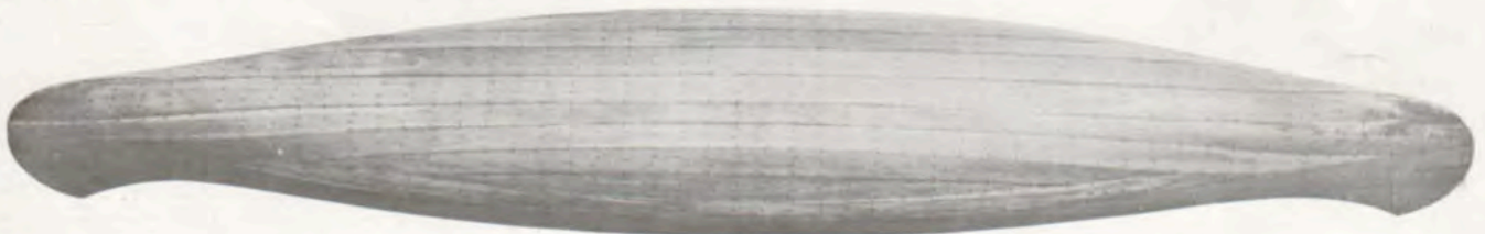
The Wooden Shell Showing the Long Length Planks in RacineWis Construction.
